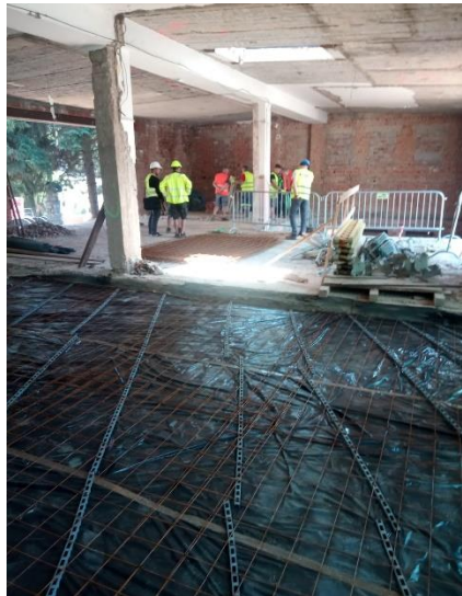
Picture 13 - Conference hall – construction works indoors...
