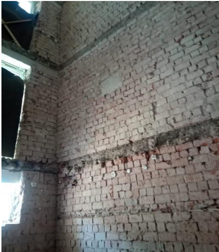
Pictures 7 and 8 - Preparation of the elevator shaft ...
